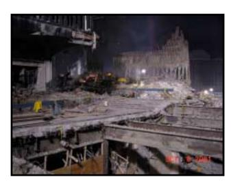
Protecting the slurry wall, which keeps out ground water and the Hudson River, is a major engineering task requiring the combined efforts of many firms. Mueser Rutledge is leading the effort, with contractor Nicholson drilling holes and placing the tie-back system that will keep the wall in place. Bovis is providing construction management. Tully is responsible for the work platforms. LiRo is helping to monitor the movement of the wall and safety of the platforms.
